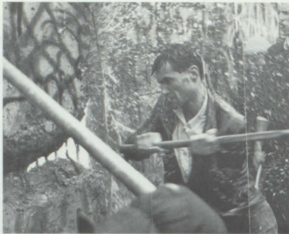
By the downfall of the Berlin Wall, West Berliners proved that the force of freedom can penetrate through the iron curtain. (Nov. 1989)
