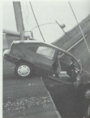
Charlestown, South Carolina was ripped apart by Hurricane Hugo. (Sept. 21, 1989)
