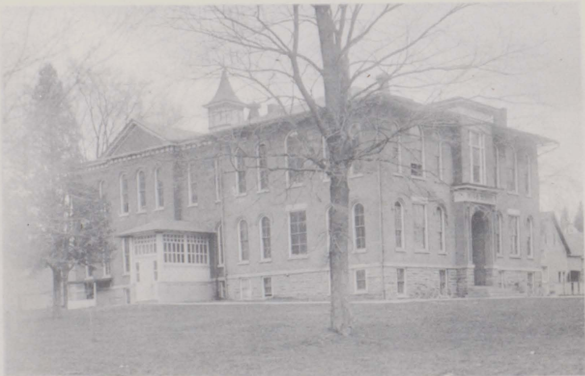
THE FIRST SCHOOL BUILT ON THE PRESENT SITE.
